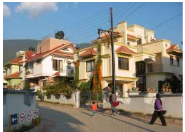
Boundary wall designed as transparent elements with short walls and grill fencing inside a housing complex in Kathmandu
