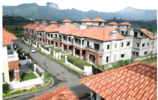
Residential Housing Complex in Kathmandu Valley
