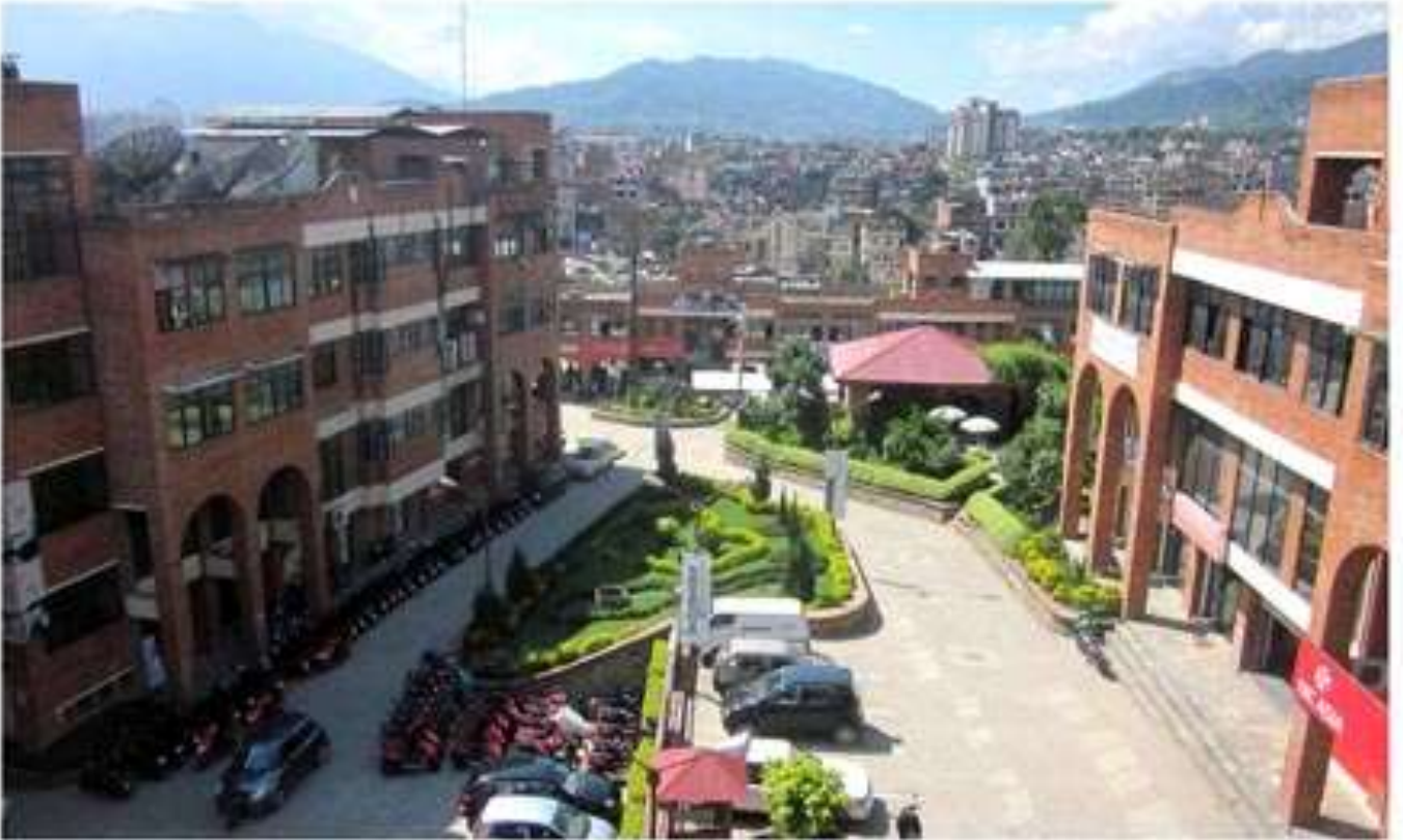
Kathmandu Business Park in Boudhabari, Teku, Kathmandu where building volumes blend with the landscape and contours of the site
