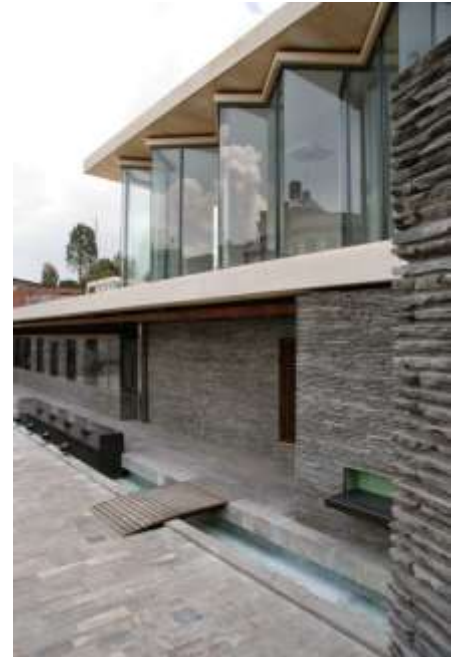
Use of exposed local stone in the Norwegian Embassy
