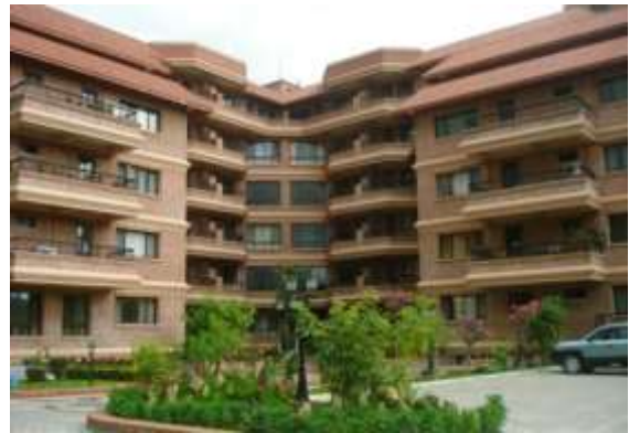
Cornices run along the façade and tie the building together in Indreni Apartments, Bhatbhateni, Kathmandu
