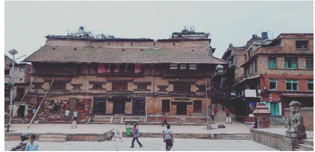
Figure 5 Front façade of Pu: Bahal viewed from Taumadhi Square.
