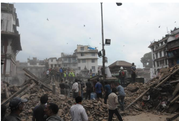
Figure 9 The ongoing rescue after the collapse of the Kasthamandap in 2015 Gorkha Earthquake Photo: Kiran Chitrakar
