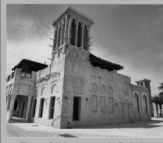
Figure 6 Windtowers in Dubai
