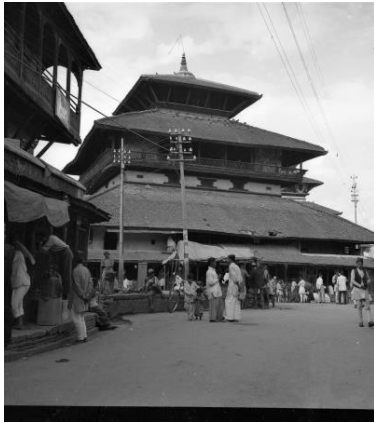
Figure 7 Kasthamandap with permanent stalls on the southern perimeter before the 1966 restoration Photo: Ganesh man Chitrakar, 1965
