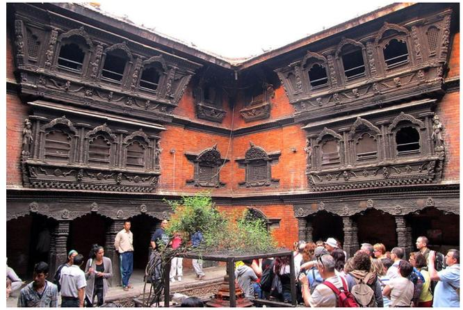
Combination of vertical columns and horizontal beams i.e. trabeated system. It consists of square based timber columns. Cornice are formed by carved timber ties. Cornice differentiate the level between three storeys. The wall (Gara) are of 24-18 inches thick which are made up of 'A' class bricks and are later on polished using varnish to give it a smooth finishing. The sculpture is three storied and is in square shaped with a chowk at middle. The chowk consists of open space.
